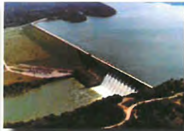
Earthen Embankment Dam
