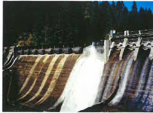
Spillway height increased by a wall of bags.
