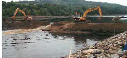
Edwards Dam being removed
