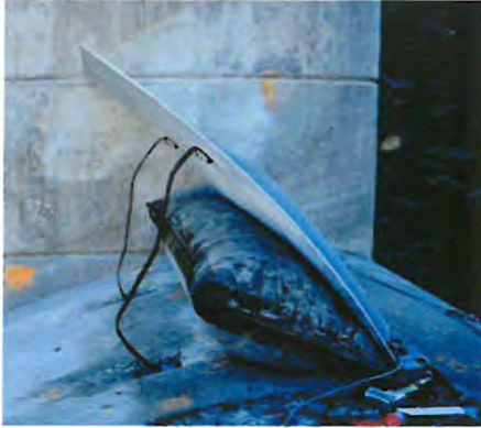
Single gate showing the bag that lifts the plate.
