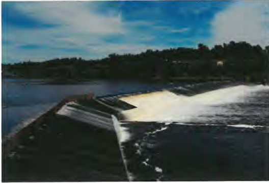
Edwards Dam prior to removal
