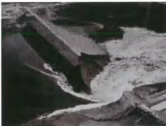
Teton Dam collapse 1976
